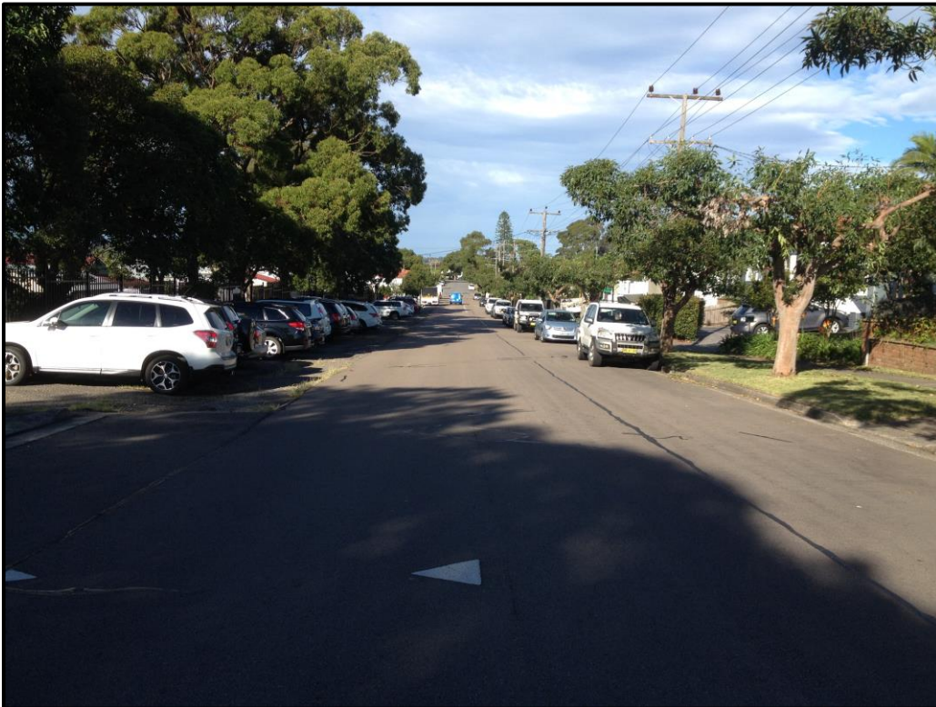
Photo 6 – View looking south along Harriet Street showing typical cross section
